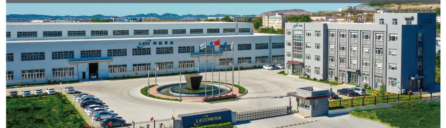
Pump Manufacturing Base for Petrochemical Industry
